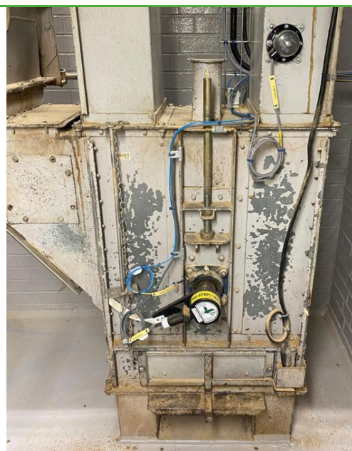
New speed, belt alignment, and bearing temperature sensors installed at the tail of an elevator
