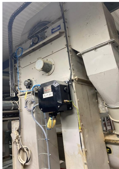
Head of an Elevator showing new belt alignment sensor, bearing temperature sensor, and junction box. You can see evidence of drum/belt rubbing causing scorch marks on the elevator casing.
